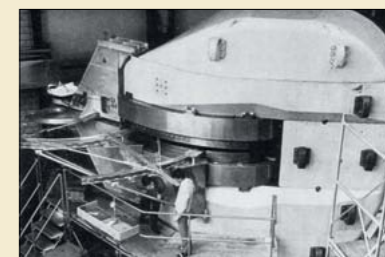
The prototype sector magnet, which confirmed that the design would provide the high-precision fields needed.
