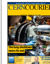
On the cover: A technician uses a mirror to inspect the positioning of the resistive soldering ovens around the last of 27,120 copper shunts that have been added to the LHC magnet interconnections, as part of the consolidation work of the first long shutdown, LS1 (p5). (Image credit: CERN-PHOTO-201404-092-28.)
