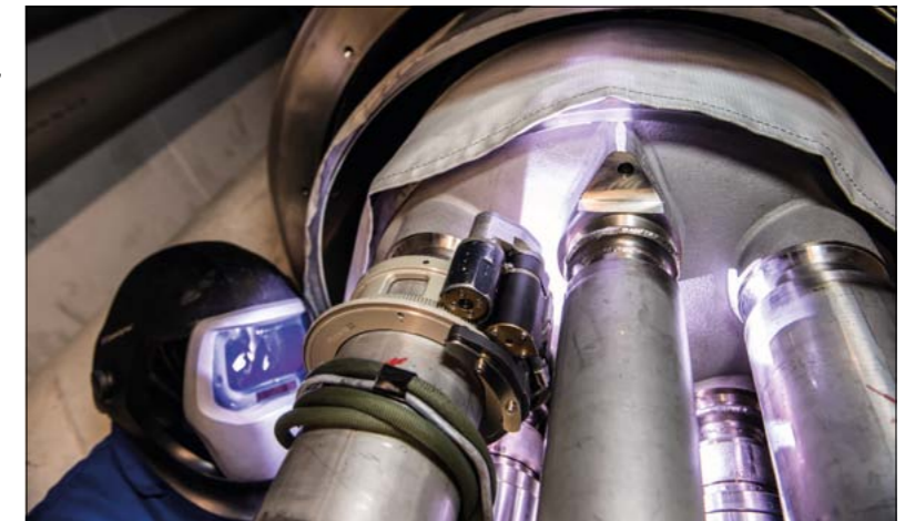
Above: By mid-April, the team welding the M-lines back together after installation of the shunts had entered the last LHC sector to be worked on. (Image credit: CERN-PHOTO-201404-084 – 6.) Right: The last of the 27,000 electrical shunts, installed on 30 April. (Image credit: CERN-PHOTO-201404-092 – 33.)
