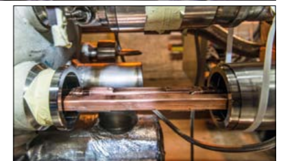
Above: By mid-April, the team welding the M-lines back together after installation of the shunts had entered the last LHC sector to be worked on. (Image credit: CERN-PHOTO-201404-084 – 6.) Right: The last of the 27,000 electrical shunts, installed on 30 April. (Image credit: CERN-PHOTO-201404-092 – 33.)
